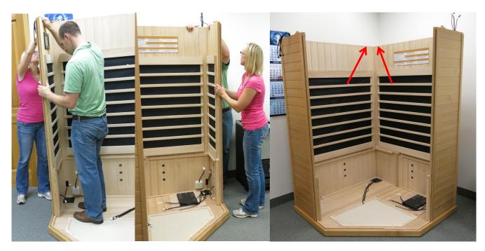
Note: When wall panels are connected in place properly the corners will be level and flush on top.
