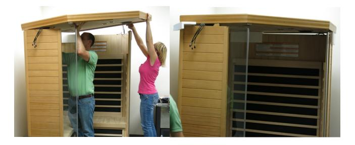
• Once the Ceiling panel is lined up directly above the Wall panels; insert the wires harnesses from the wall panels into the holes in the Ceiling panel.
