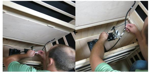
• Locate the electrical switch on the black Master Control Box and ensure the switch is on.
