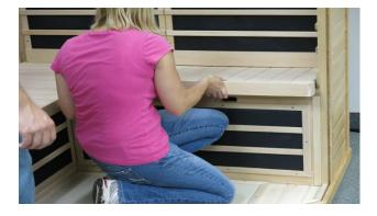
The Bench Top should fit down flush from front to back. It may be necessary to use the
