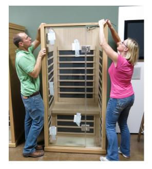
**Note:** Secure the door from falling open and breaking while setting the Front Wall panel. It may be helpful to use your knee to help push in the Front Wall panel while lowering into place.
