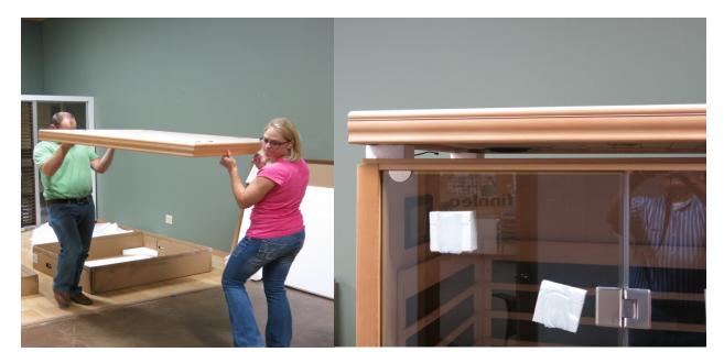
• Once the Ceiling panel is lined up directly above the Wall panels; insert the wires harnesses from the wall panels into the holes in the Ceiling panel.
