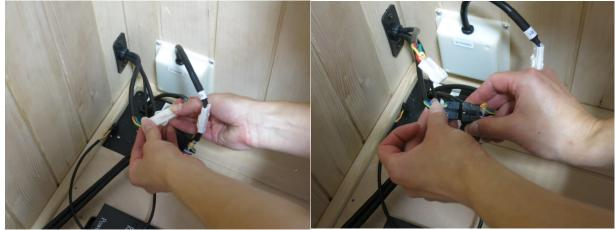
• Connect wire R1 from the distribution plate to R1 from the Right Wall junction box.
