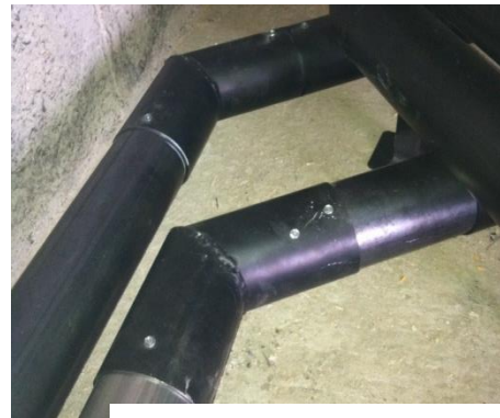
Securing the tube in the socket with self-tapping screws.
