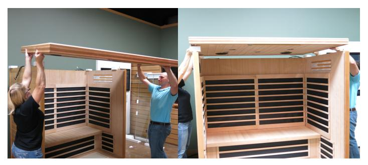
• Once the Ceiling panel is lined up directly above the Wall panels; insert the wires harnesses from the wall panels into the holes in the Ceiling panel.
