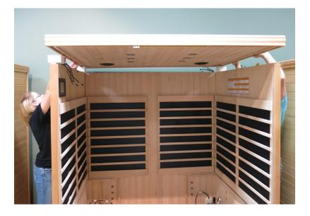
• Once the Ceiling panel is lined up directly above the Wall panels; insert the wires harnesses from the wall panels into the holes in the Ceiling panel.
