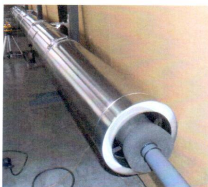
Photo 3. Course of gas tightness test of SKDTŻ-3L chimney using a Wöhler unit
