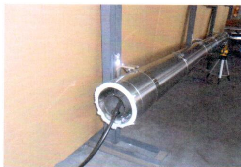
Photo 2. Sealing of the chimney system during gas tightness test.
